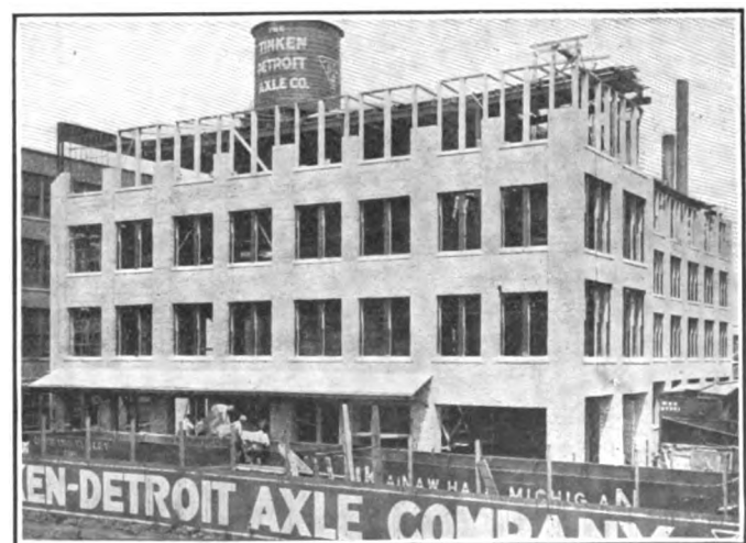
Timken-Detroit Axle Company's new plant, now under construction
